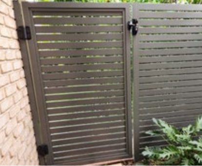
Aluminium slat fencing and gates
