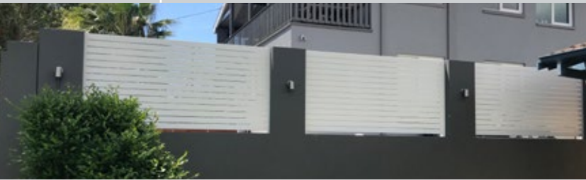
Aluminium slat brick pier infills
